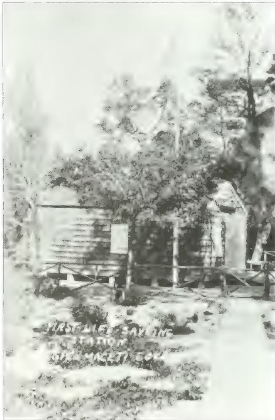
Figure 2.4. Spermaceti Cove Lifeboat Station, circa 1930. In 1849, the U. S. Treasury Department's Revenue Marine Board established a lifesaving station at Spermaceti Cove to protect mariners along the southern portion of Sandy Hook (U. S. Coast Guard, "Station Spermaceti Cove, New Jersey," http://www.uscg.mil/history/stations/SPERMACETICOVE.pdf ).
